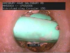
Underground drainage pipes can be damaged by public utilities works as well as tree roots and silt
